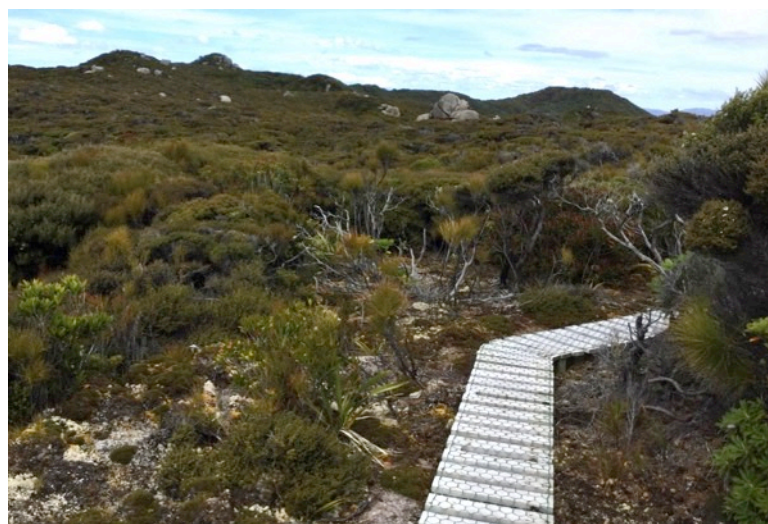
Part of the boardwalk, installed to protect the low vegetation and make for easier and faster access.
